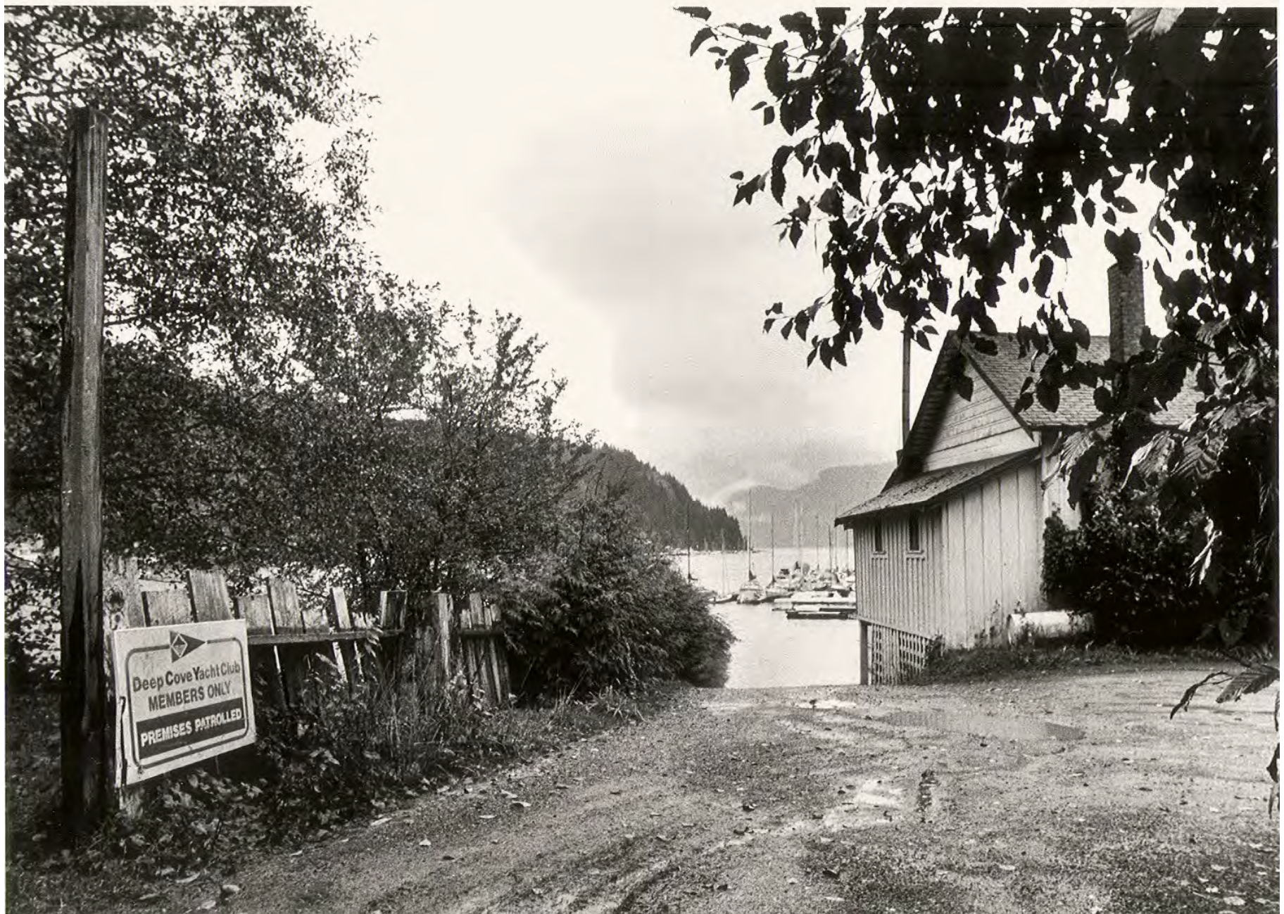
The club parking area and access to the ramp.
