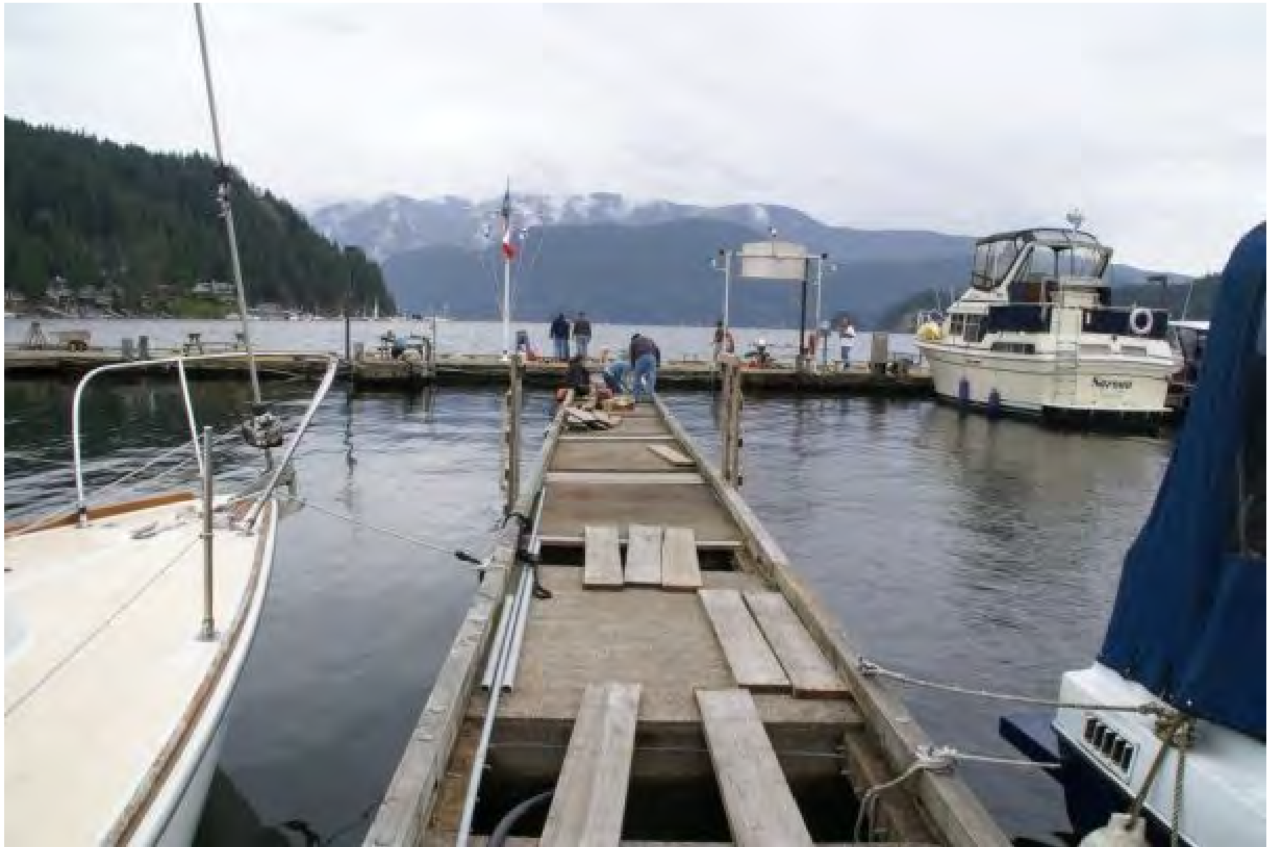
The crew adding 45 feet to the walkway.
