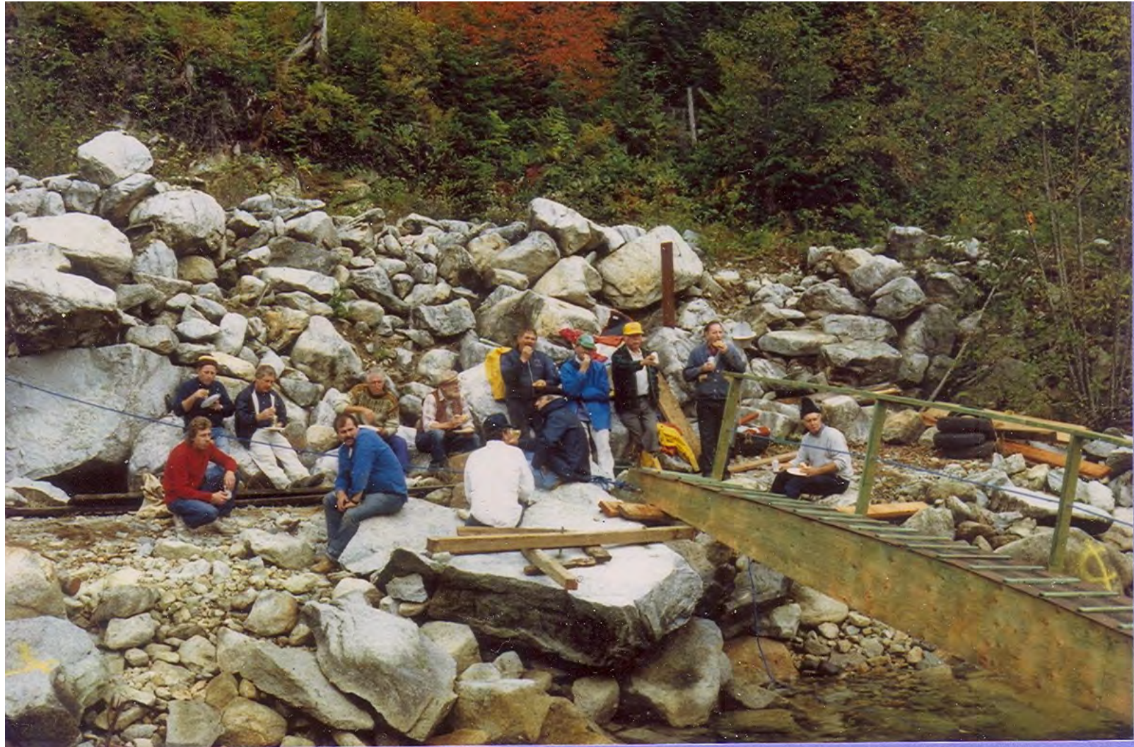
With the ramp temporarily in place, the crew take a break.
