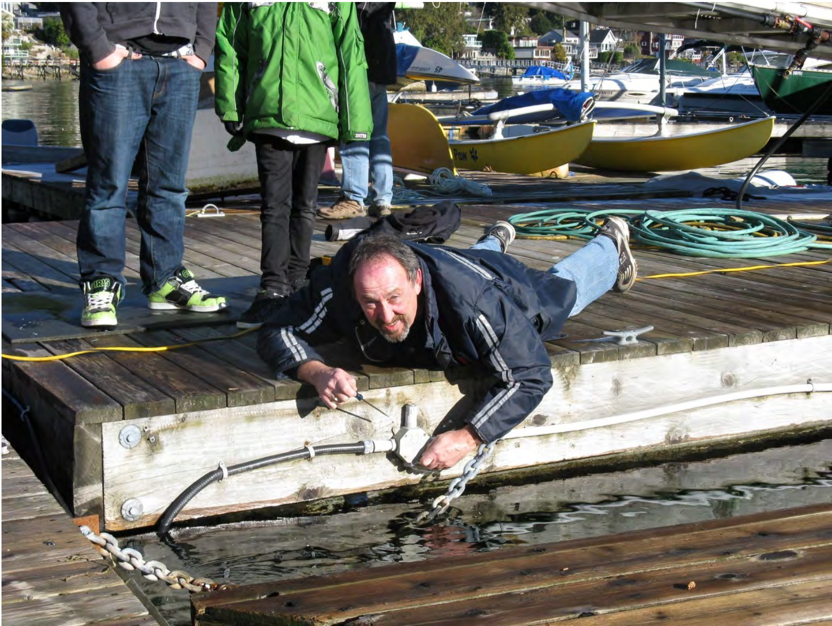
Commodore Mark Doucette disconnecting the electrical distribution system.
