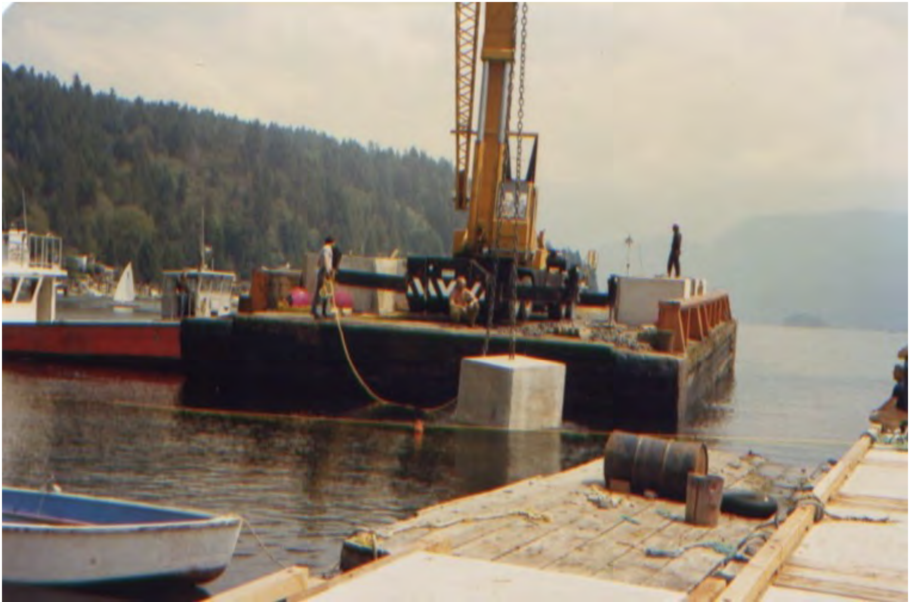
A 12T block being carefully lowered on 7/8" long link chain.
