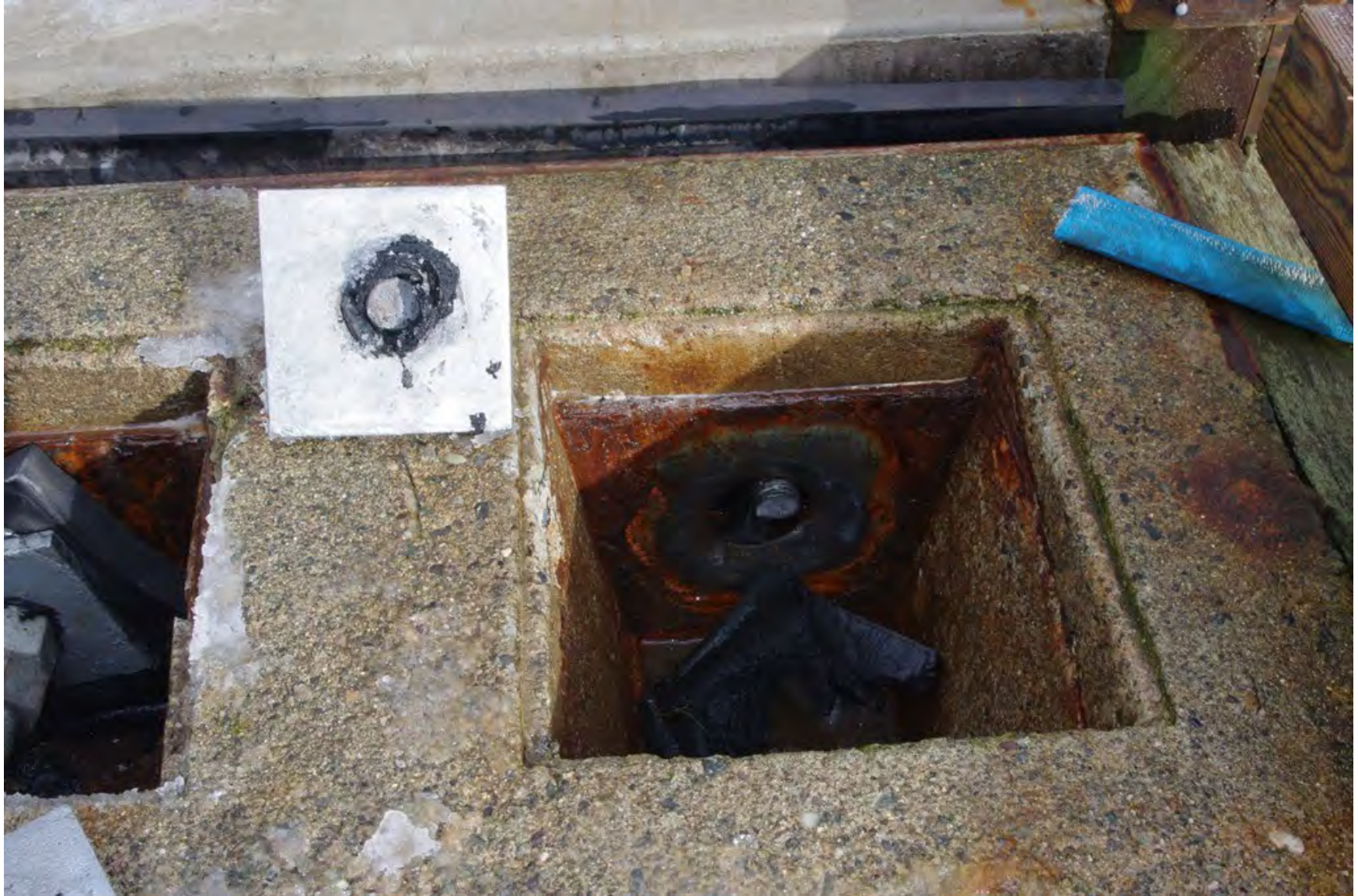
A failed connector bolt on the new section of A Dock, during the winter of 2010/2011
