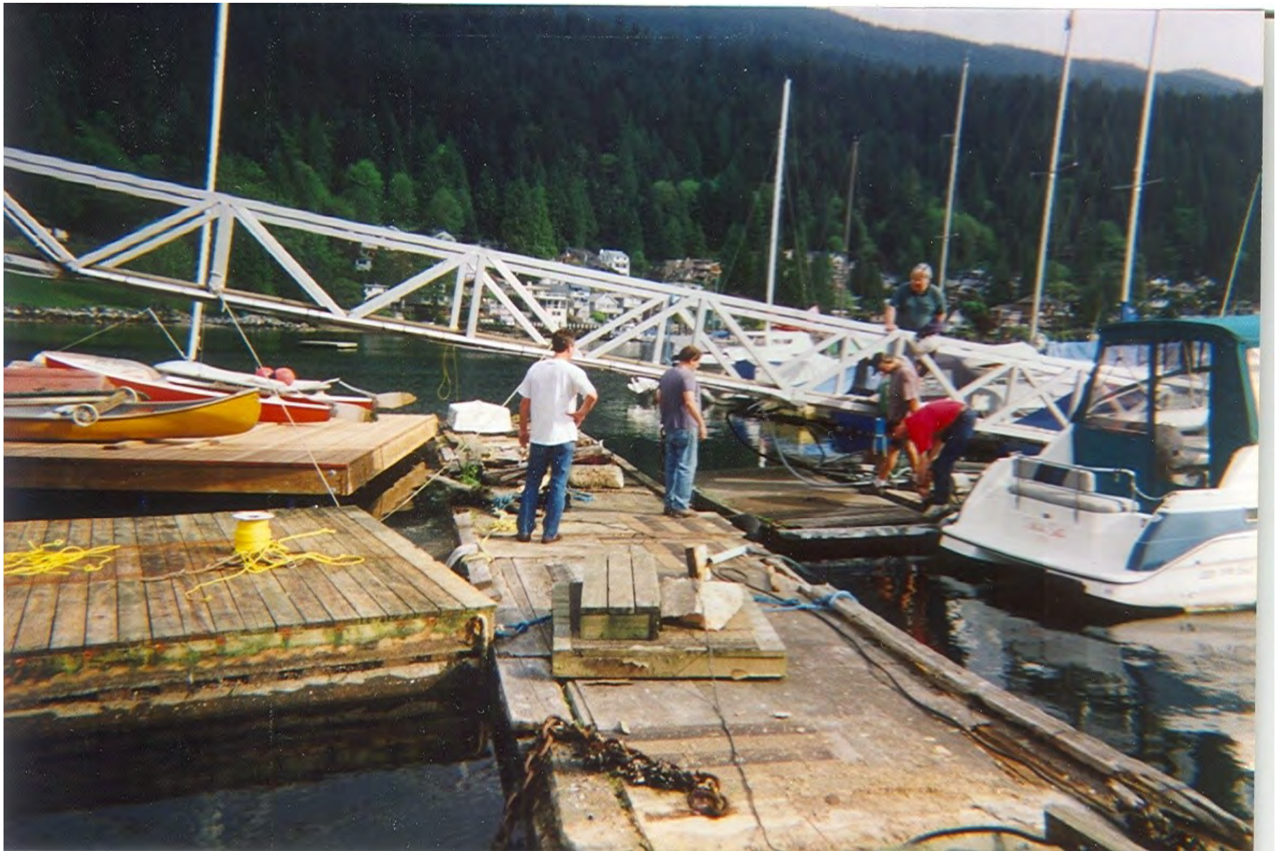
Maneuvering the dock under the ramp. The old log dock can be seen in the foreground. It is about to be relocated and the new dock moved into place.
