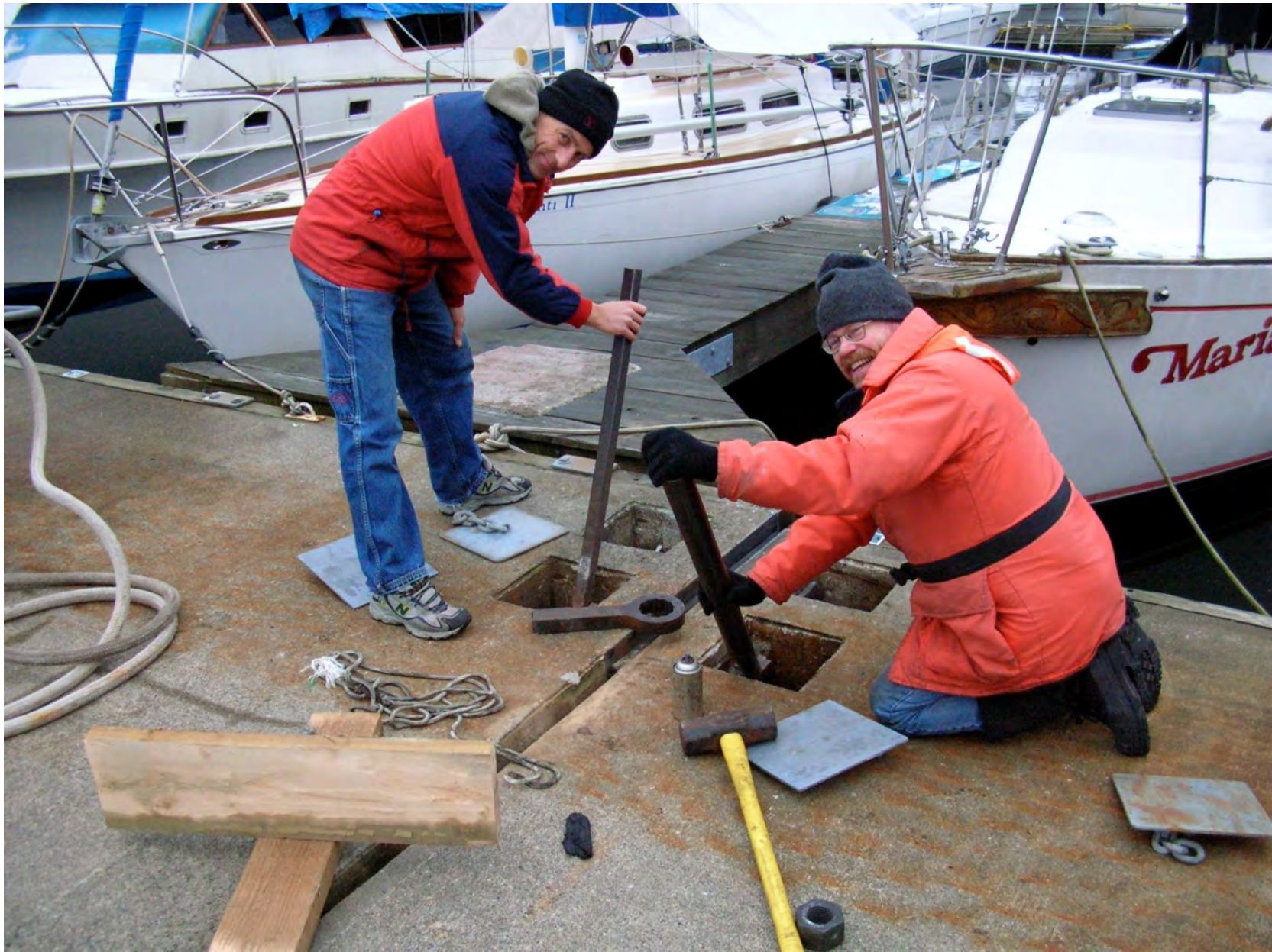
Tony Gill and Doug Hill tightening the connector on A Dock
