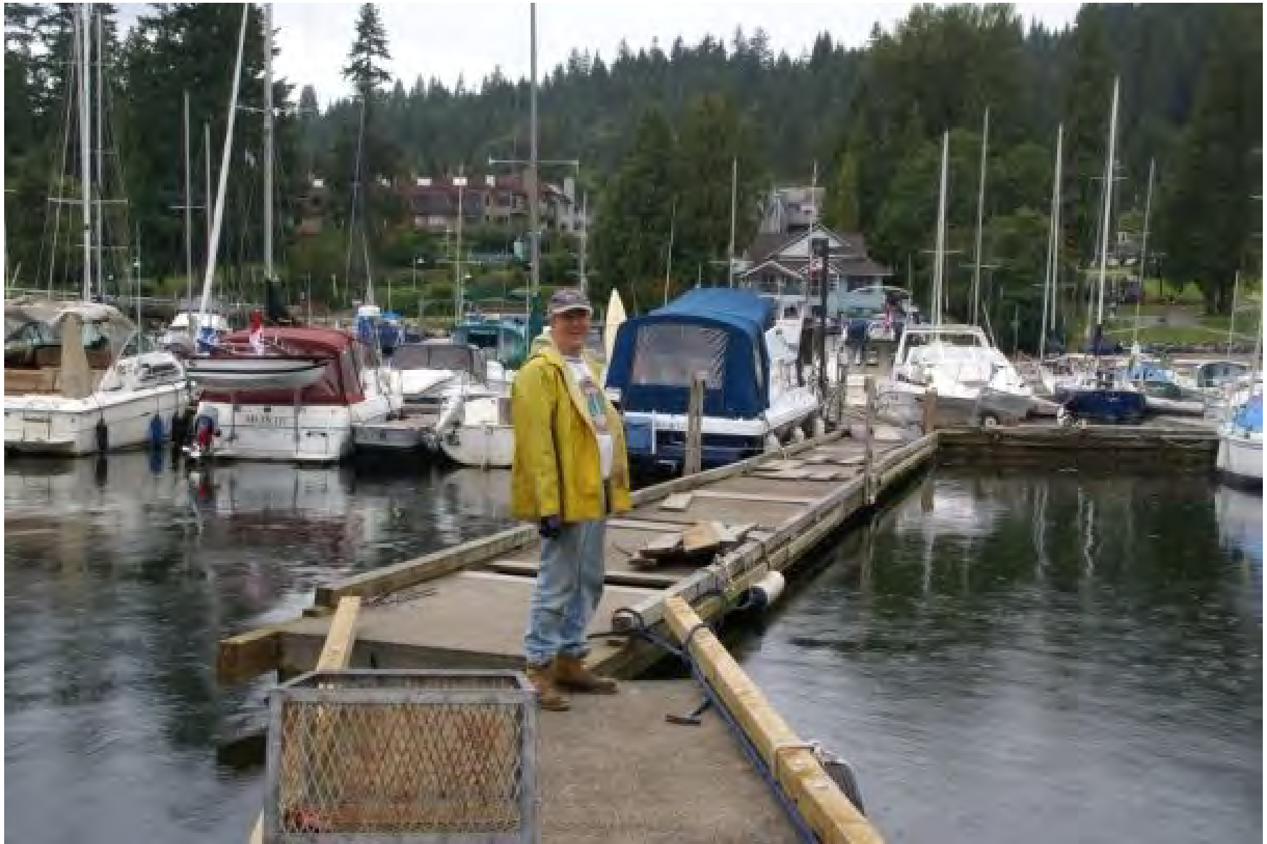
Working on disconnecting the main walkway prior to inserting the extension.
