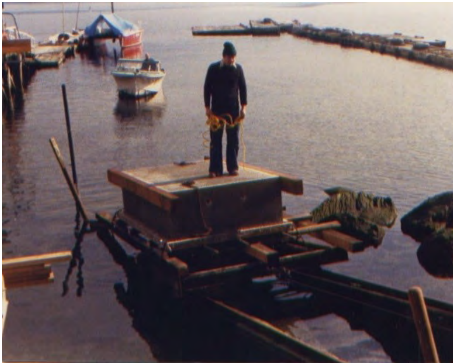
Launching the first concrete module for the main walkway. The units were constructed by club members on a marine railway right next to the old club house. Spring 1980.
