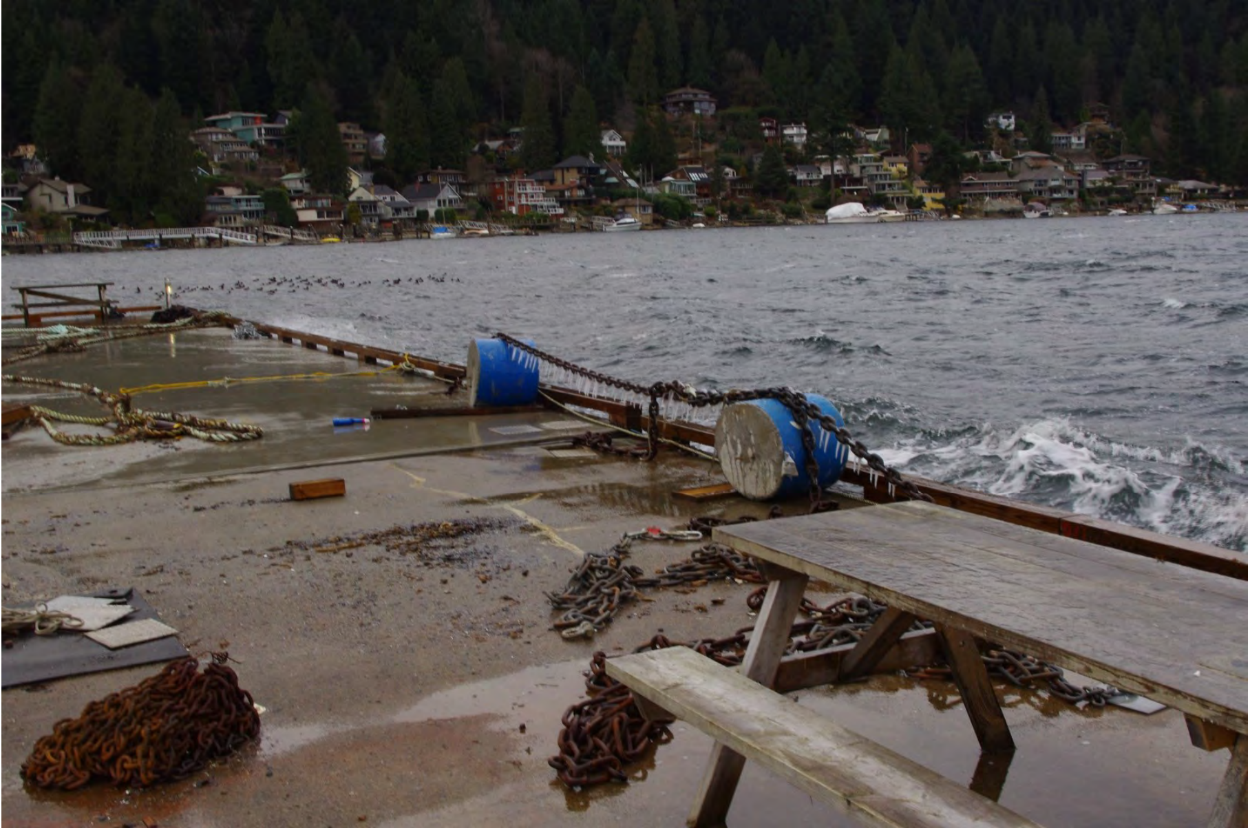
A temporary fix.
