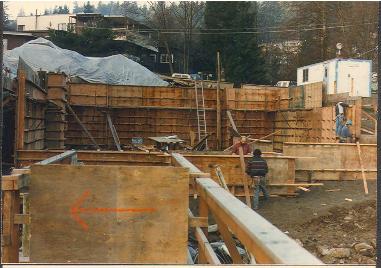
The forms for the basement concrete foundations January 1985.
