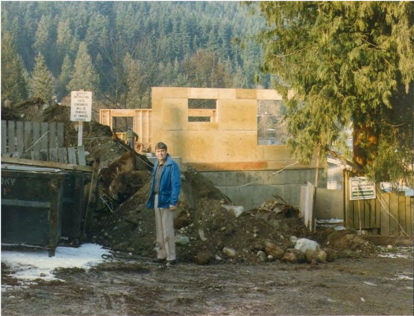
The main floor framing progressing under the watchful eye of Keith Byers – February 1985.
