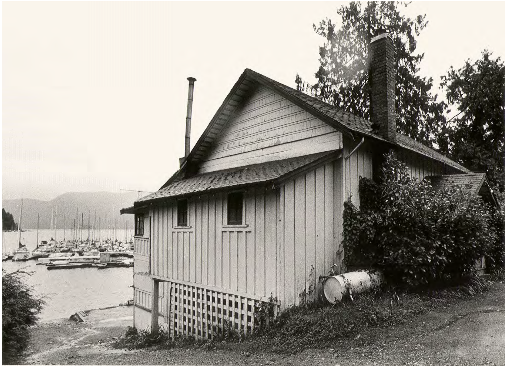
The north side of the building looking down the ramp to the water. From a small unpaved parking area in front of the club house.
