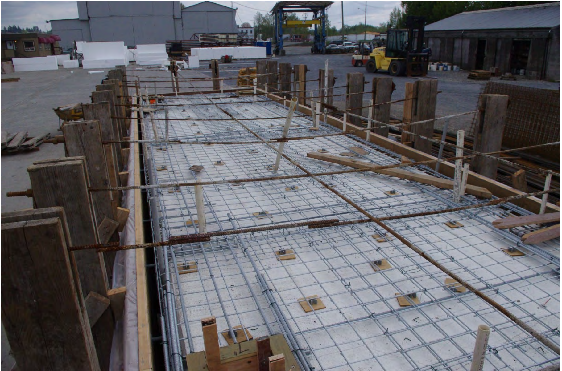
A check of the extension sections for B and C Docks during construction
